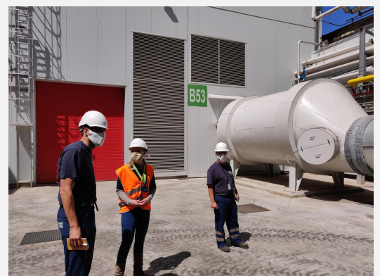
Lien Van Schepdael, Technical Account Manager at Flexcity, next to the gas turbine of Beneo Orafti Oreya and with Guillaume Poncelet, Power Plant Engineer at Beneo.
